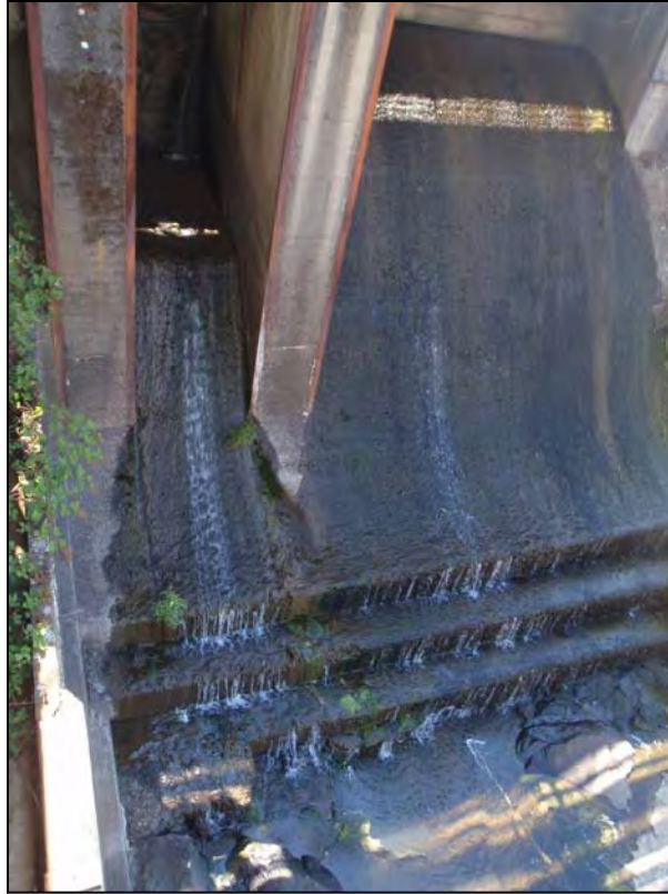
Photo 15. Flashboard weir on the PGE dam (08/03/2012).
