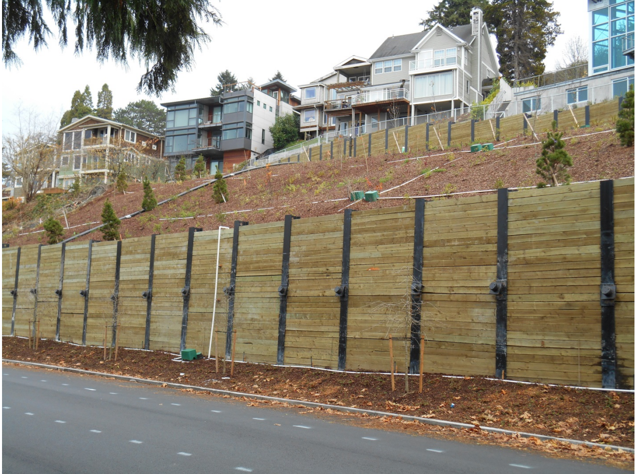
Sample Soldier Pile and Tieback Retaining Wall with Wood Lagging
