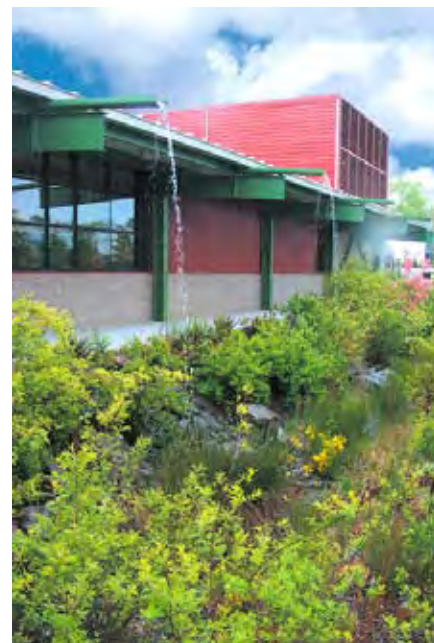
Capturing stormwater run-off from buildings in landscaped swales
