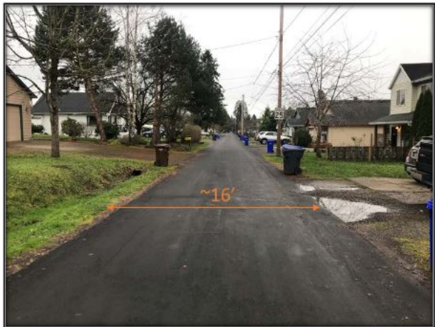
Figure 2-5: Narrow Roadway (Hiram Ave)
