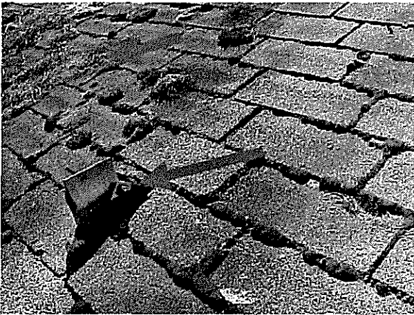
Poor roof shingle condition with moss build up and old hardware penetration through the shingles.
