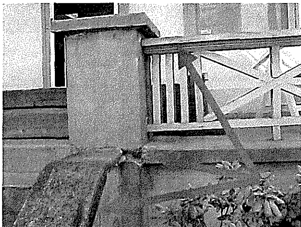
Rotted railing at the front porch. Cracked and chipped concrete At the stairs and pillars.
