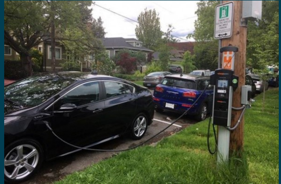
PGE on-pole charging in SE Portland
