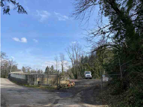
City Maintenance Yard
