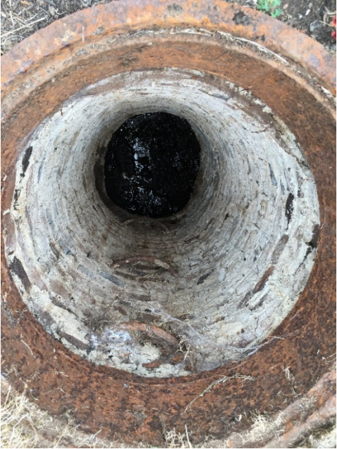
Figure 4-1. Historic brick manhole along the Singer Creek alignment
