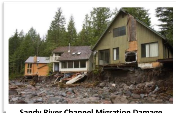
Sandy River Channel Migration Damage January 16, 2011
