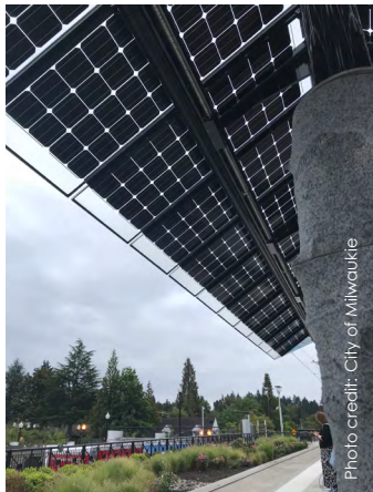
Solar panels at MAX Station
