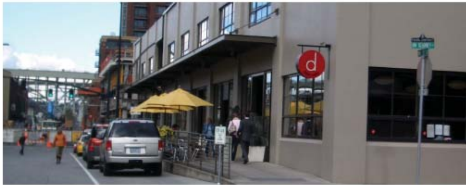
Figure Xc. Retrofitted industrial building with horizontal awnings.
