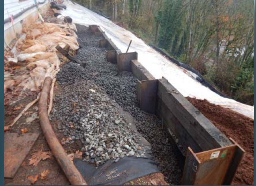
Geotextile fabric and drain rock placed in the benched excavation behind Bays 12 through 18
