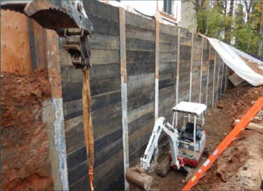
Lagging installation from Bay 1 through 11
