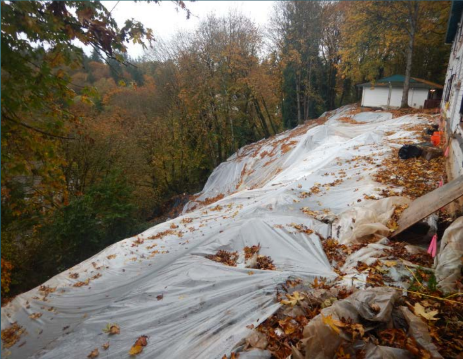
Plastic sheeting covering the slope downhill from the duplex and 8-Plex
