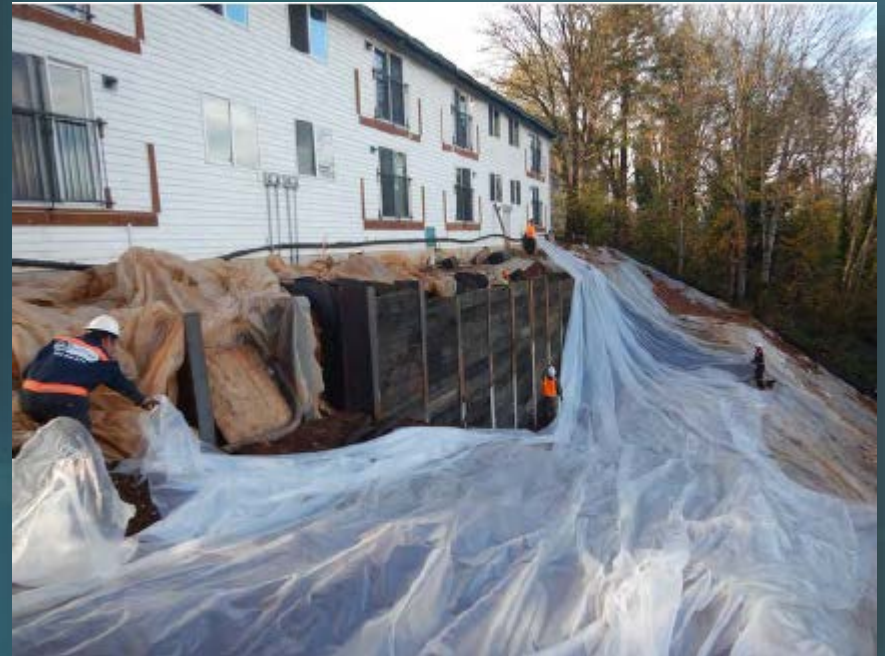
Plastic sheeting installation over excavated area near lagged retaining wall
