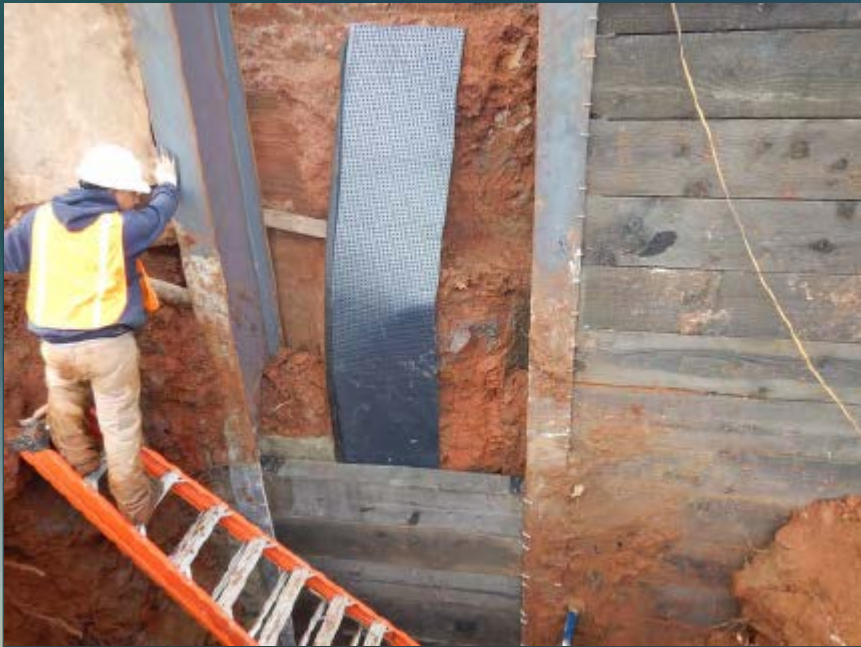
Personnel installing lagging and drain board for Bay 18
