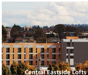
Central Eastside Lofts
