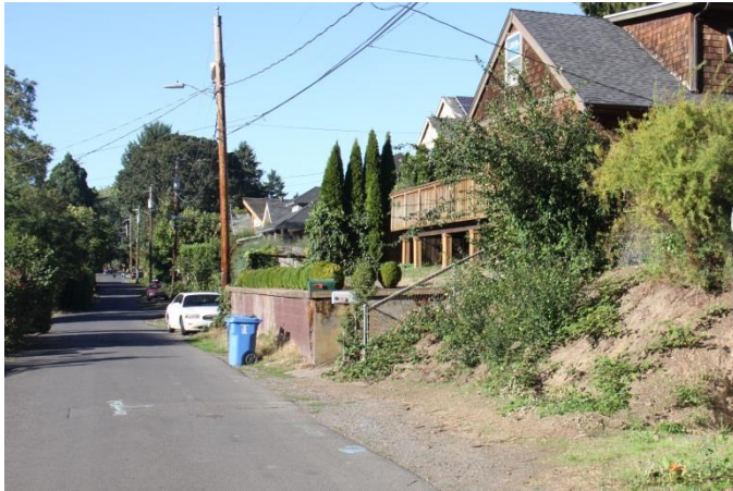
The elevation increases rapidly on the east side of the street (right side of photo) limiting the ability to widen the roadway
