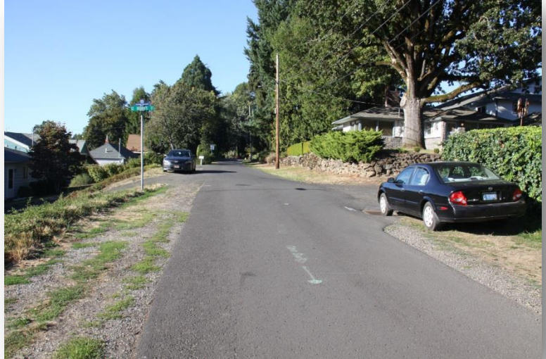
SE 19 th Avenue: Looking north Unpaved shoulders are often landscaped or used for parking. Also note the rapid drop-off toward the river (left side of photo) that constrains the right of way
