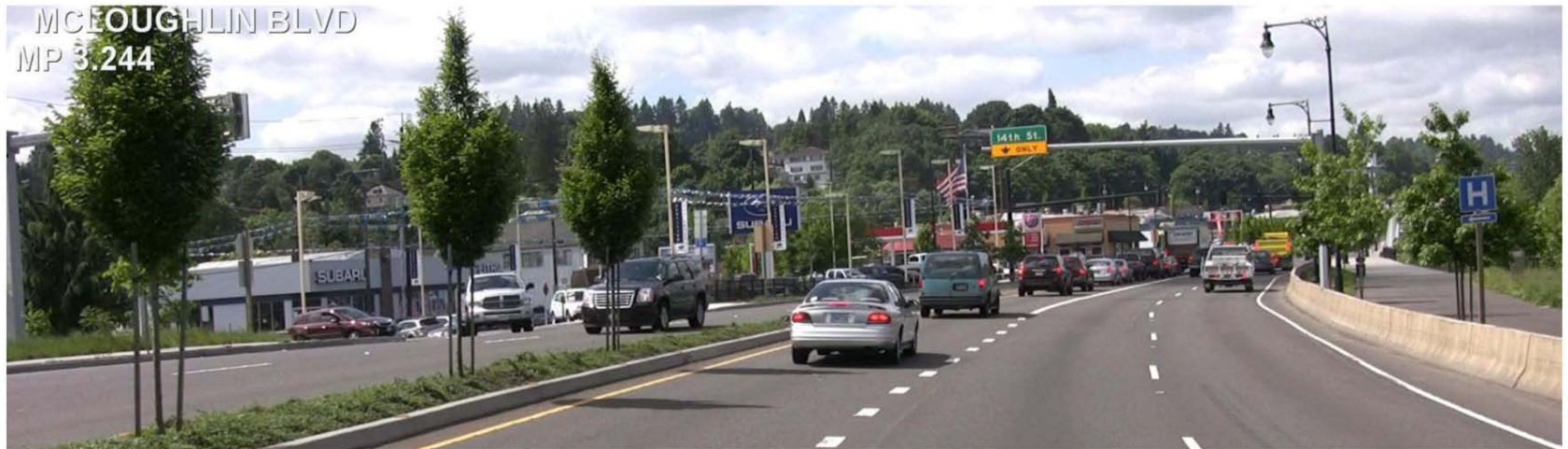
Looking south on McLoughlin Boulevard at the I-205 interchange northbound on-ramp
