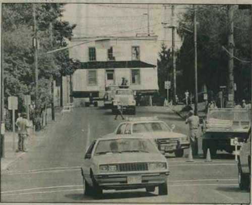
The Ermatinger House starts an uphill trip. Winching cables were used at this point of the transfer to move the structure.
