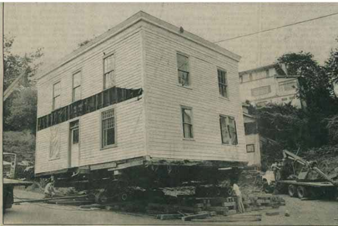
Raised on a platform called cribbing, the Ermatinger House is prepared to make the journey to a new location near 6th and John Adams. Built around 1845, it is the oldest house in Oregon City.
