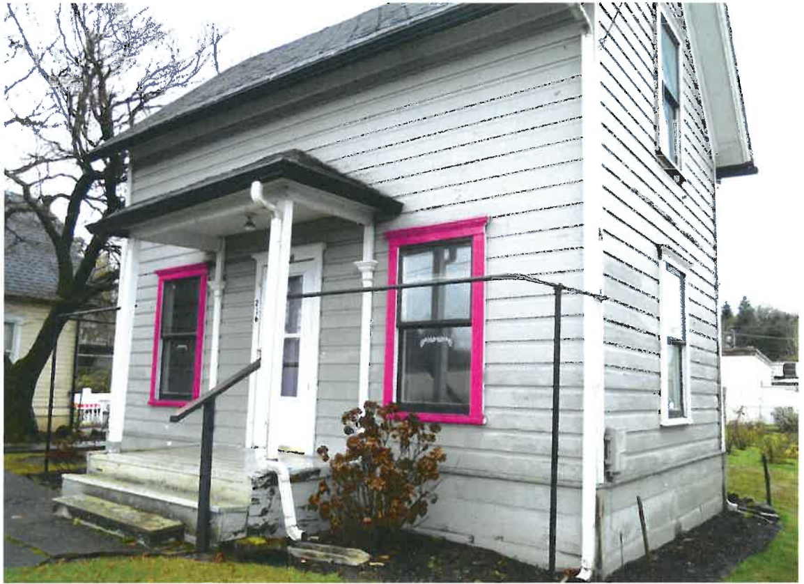
View of Property looking South
