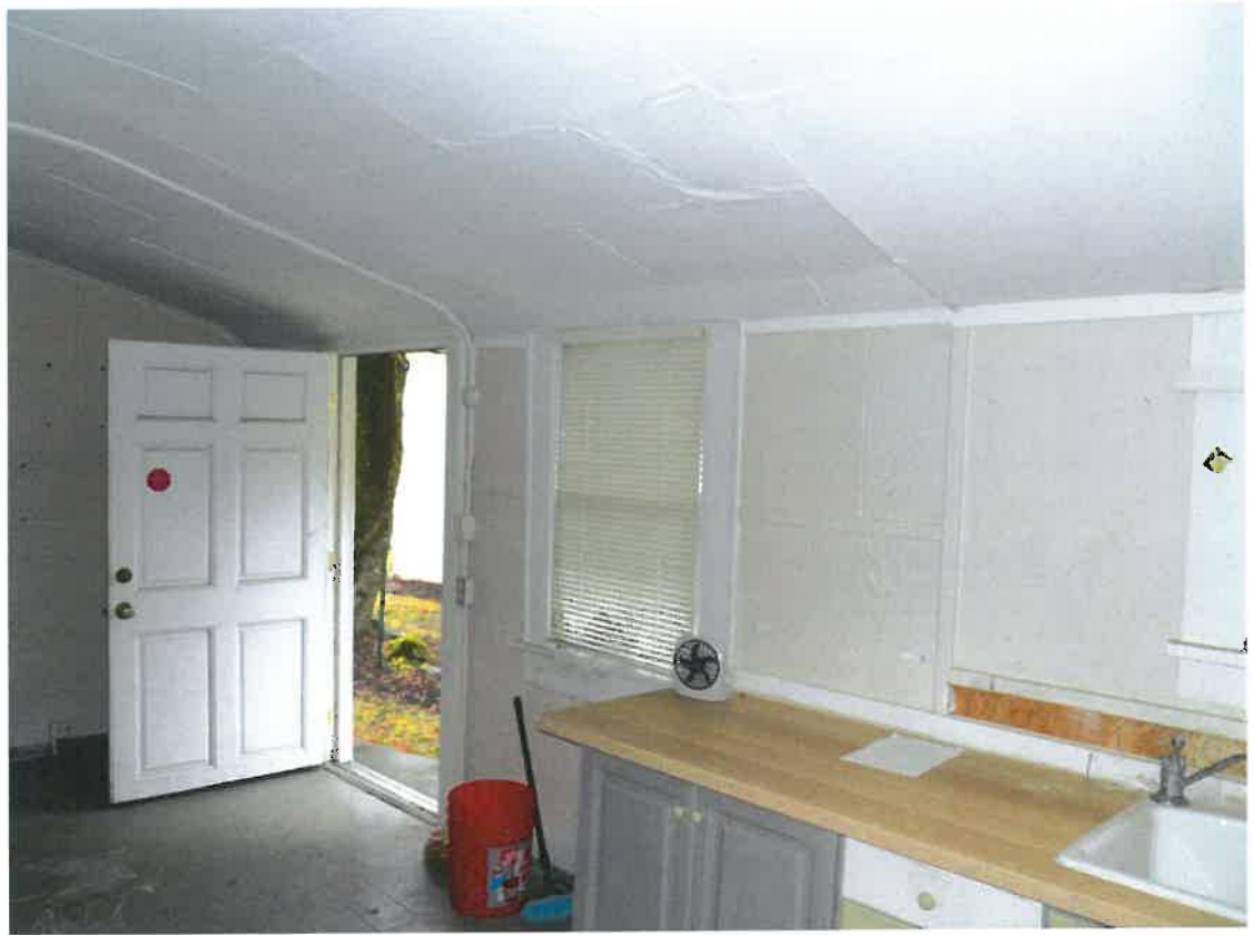
View of Existing Side Entry (Kitchen)
