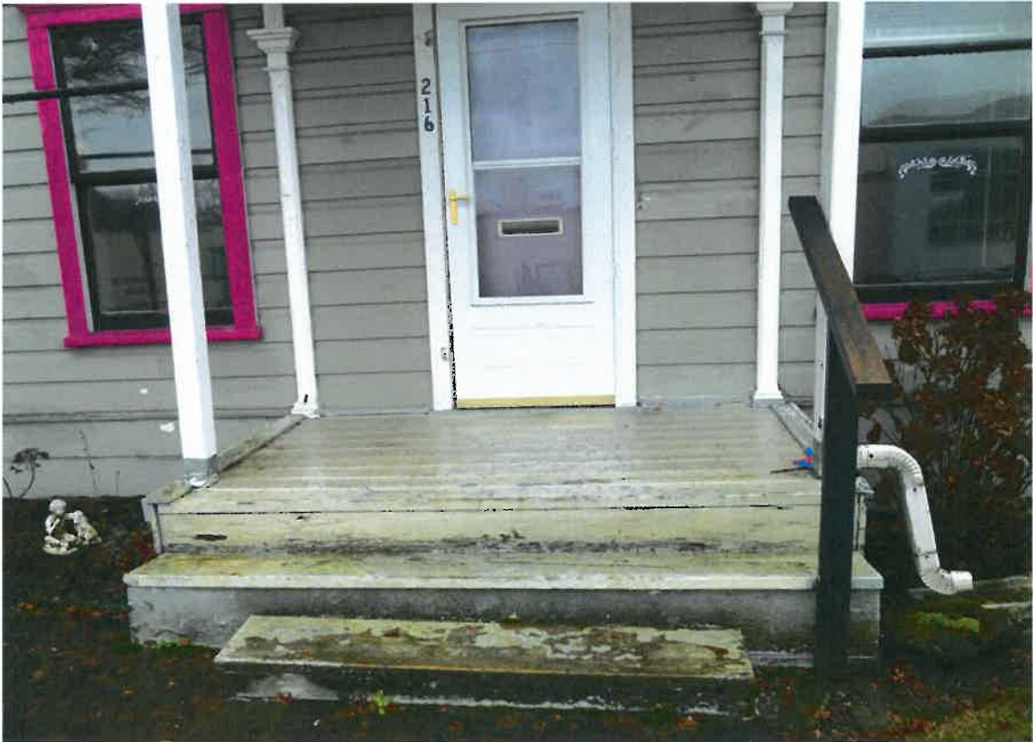
View of Existing Front Entry and Porch
