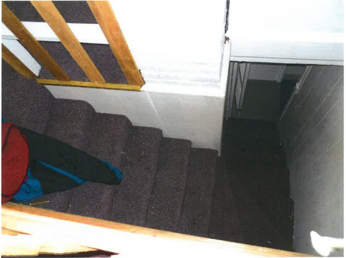
View From Upper Level to Main
