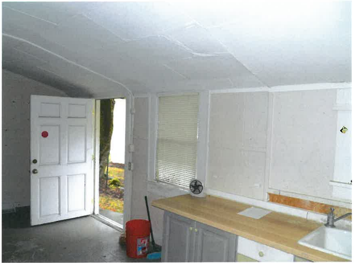
View of Existing Side Entry (Kitchen)
