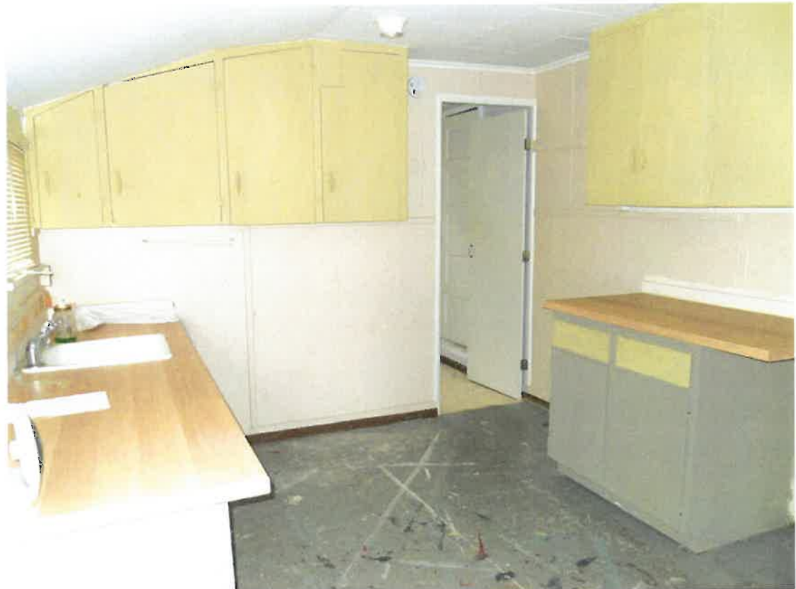
View of Existing Kitchen
