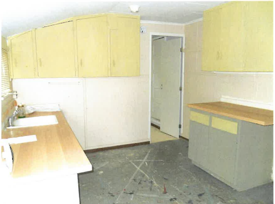
View of Existing Kitchen
