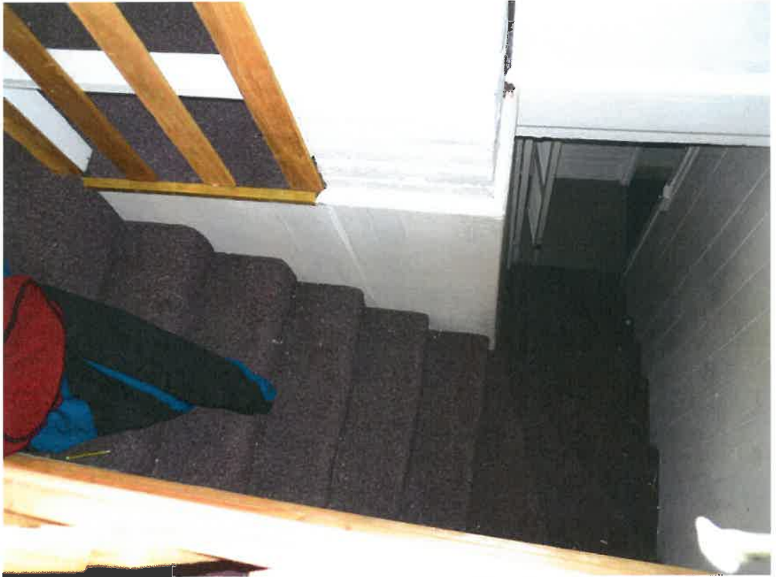
View From Upper Level to Main
