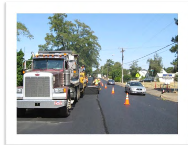
Pavement overlay on South End Road
