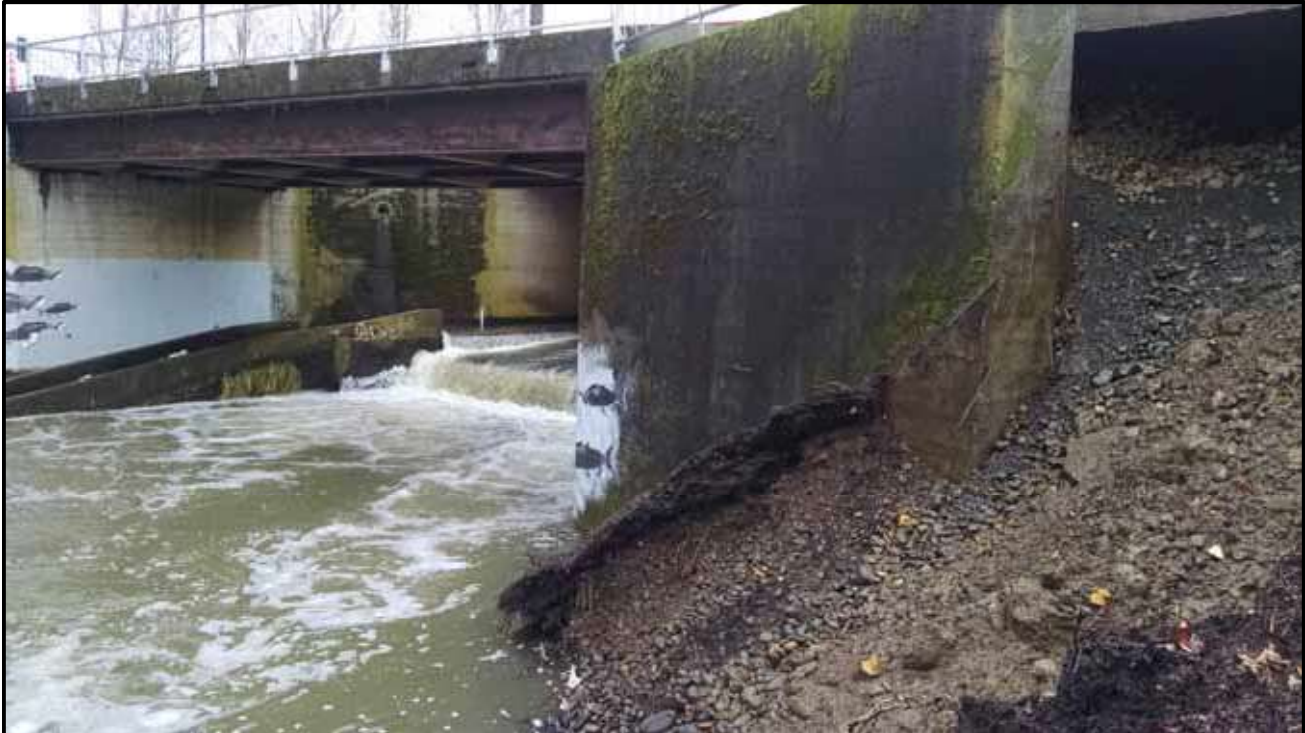
Slope below bridge
