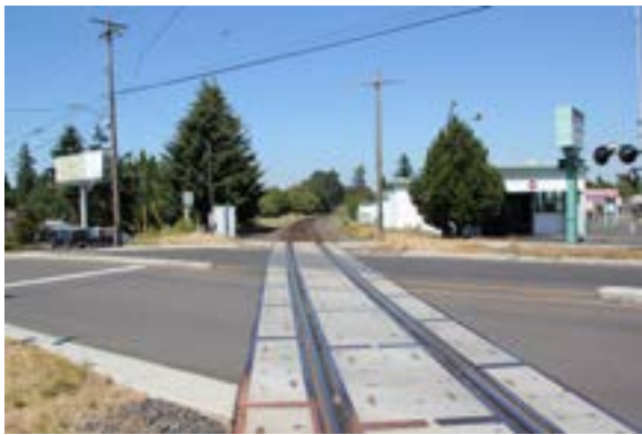
The railroad crossing at SE Harrison St requires improvements to increase pedestrian safety.
