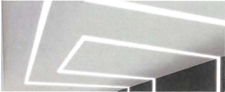
RECESSED LIGHTING AT SOFFIT
