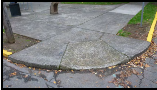
Figure 6: Share Curb Ramp at NE corner of John Adams and 6 th Street
