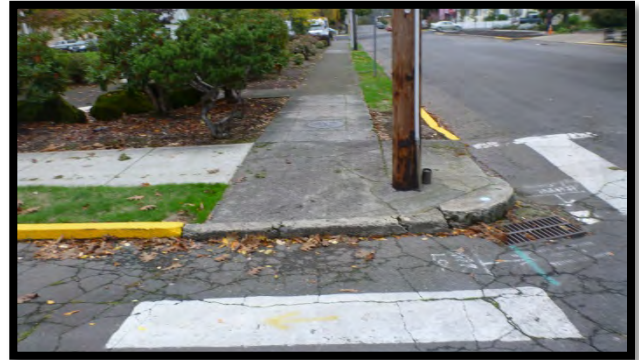
Figure 7: Missing Curb Ramp at SW corner of John Adams and 6 th Street
