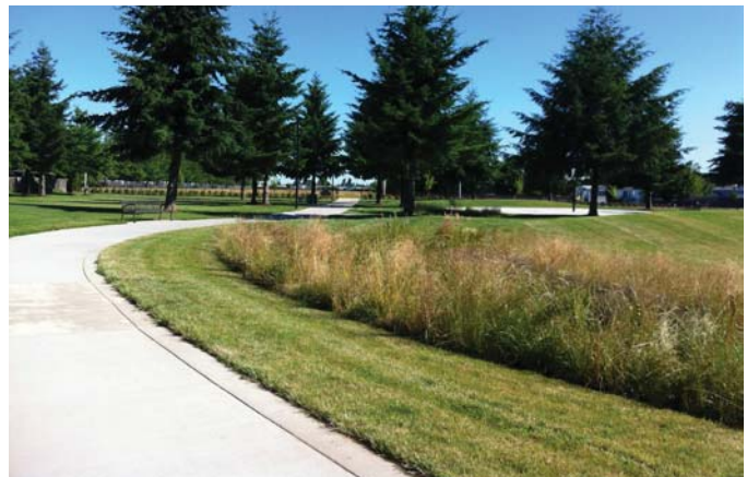
Example of a multi-use pathway at grade
