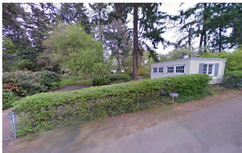
Figure 2. Existing Conditions – street view
