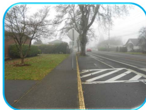
Midblock crossing at former Mt. Pleasant School
