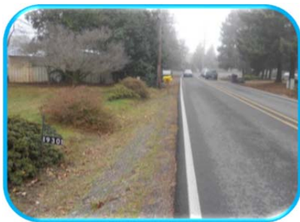
Shoulder and ditch on Leland Road (Segment 3)
