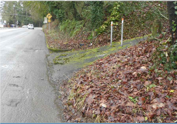
Path connection at 5th Street has no wayfinding signage. In addition, lack of landing and steep slopes are a hazard for path users.
