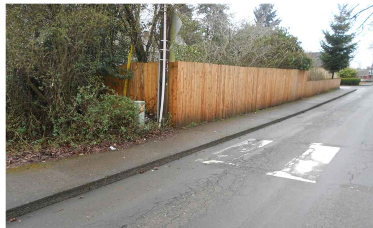
Crosswalk from neighborhood lacks sidewalk landing
