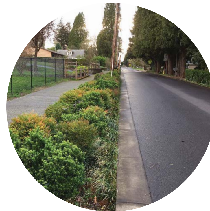
The nearby Logus Road project incorporates stormwater treatment and traffic calming features
