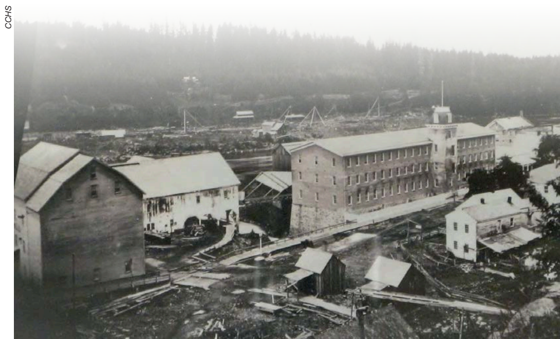
1870 Woolen Mill along Main St. The Mill's foundations remain.
