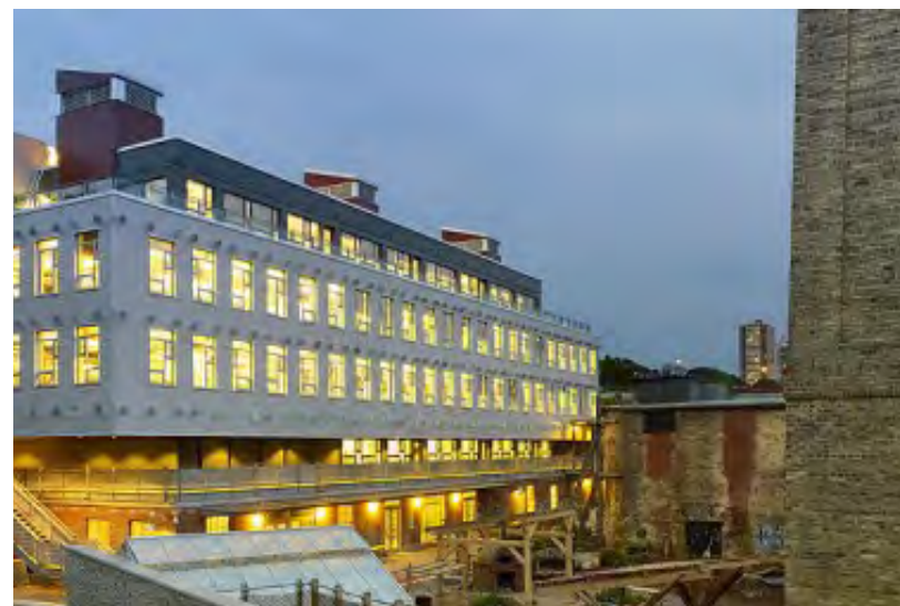
New construction at Evergreen Brickworks, a community center and non-profit organization in Toronto, Canada.
