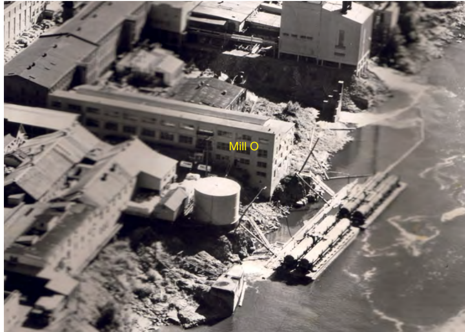
Mill O extends west from Main Street and the Woolen Mill in this 1955 photo.
