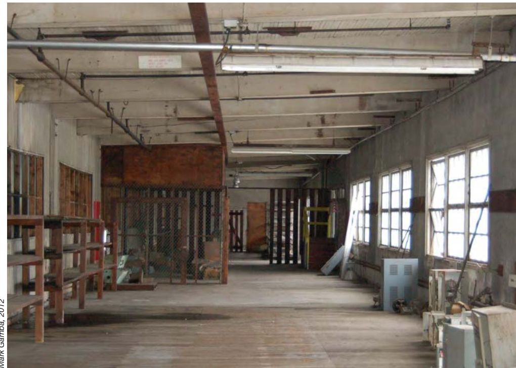
In addition to the massive concrete column and beam mill structures, wood framed buildings exist on site with exposed wood columns, beams, and roof trusses. A renovated Mill O could be a unique space with distinct character.
