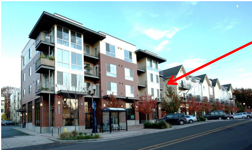
Figure 4. Significant break in building façade. This break is a physical separation
