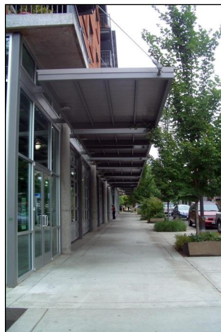
Figure 7. Canopy with balcony incorporated.
