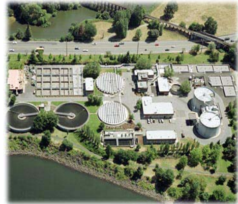
The Kellogg Creek sewage treatment plant is located west of McLoughlin Road in Milwaukie along the Willamette River.
