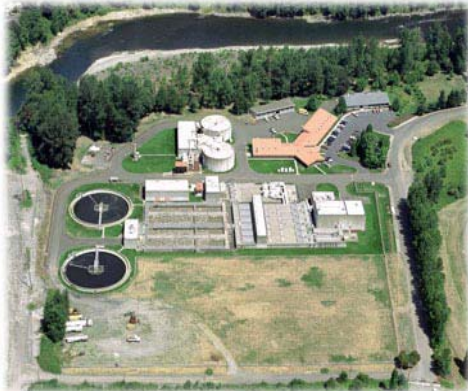
The Tri-City sewage treatment plant is located west of the I-205 Park Place exit near the Clackamette Cove.
