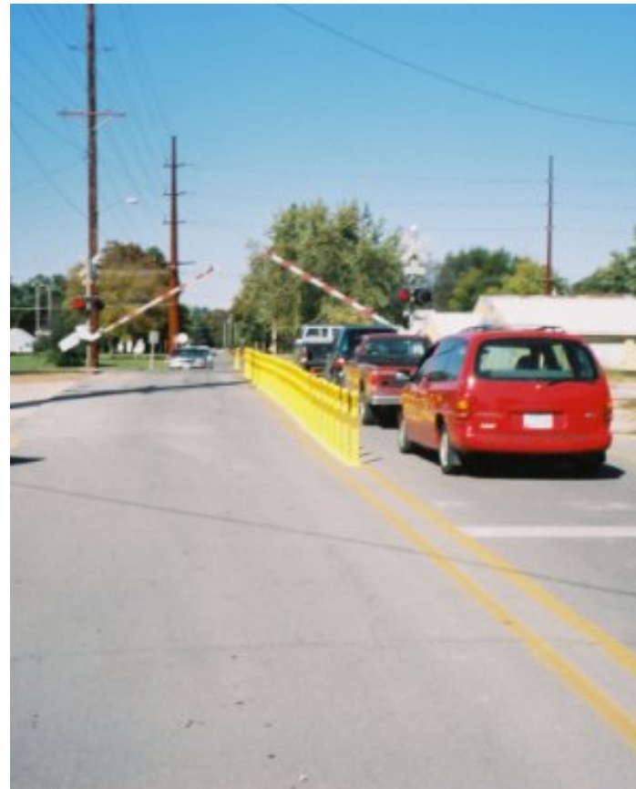
Median barrier SSM with existing gate arms.
