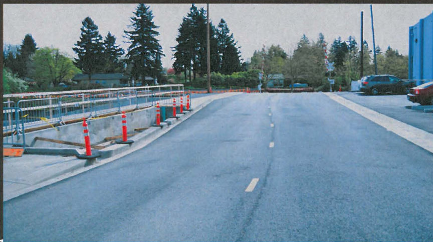
Mailwell west of the rail with new sidewalk and stormwater planter
