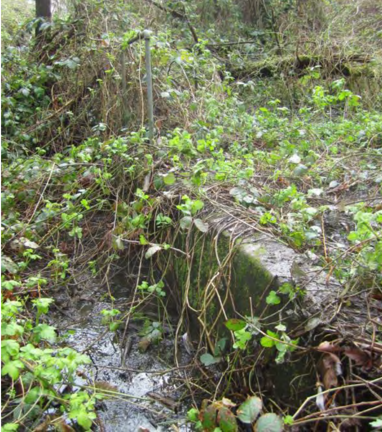
Photo 4. The remnant concrete wall.
