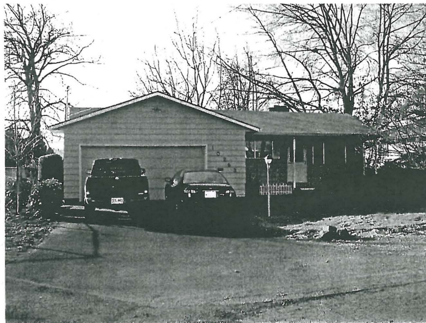
View of PMH building from SE 36th Avenue.
