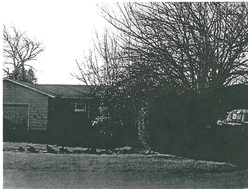
Side yard on north side of PMH building.
