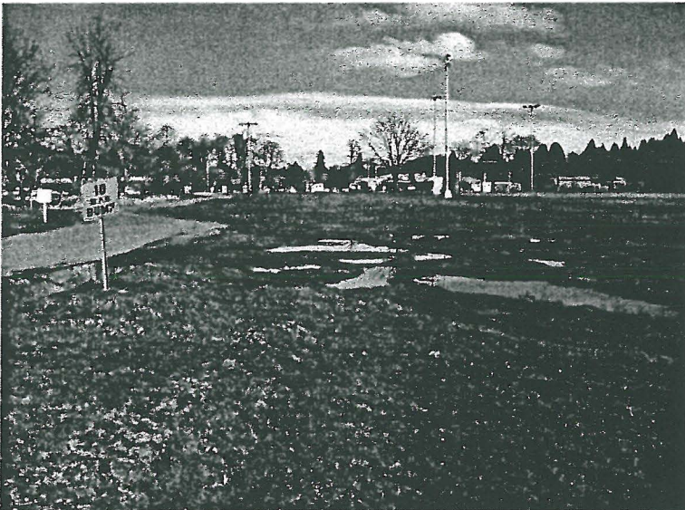
Photo B showing water ponding on fill in Wetland 1
