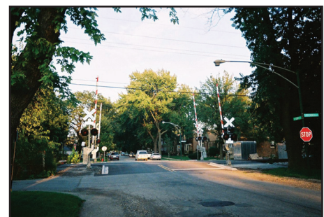
Four quadrant gates at a crossing in Illinois
