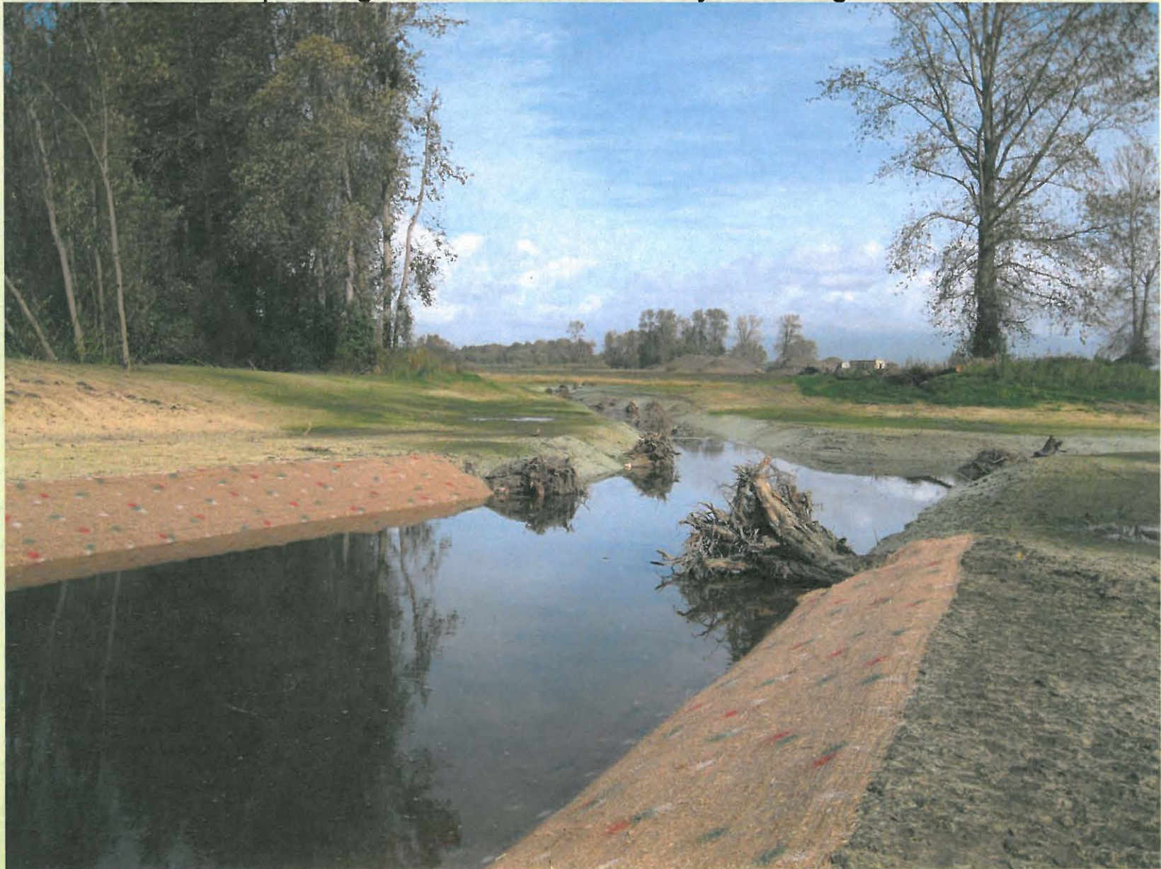
Nookachamps Mitigation Bank immediately following construction
