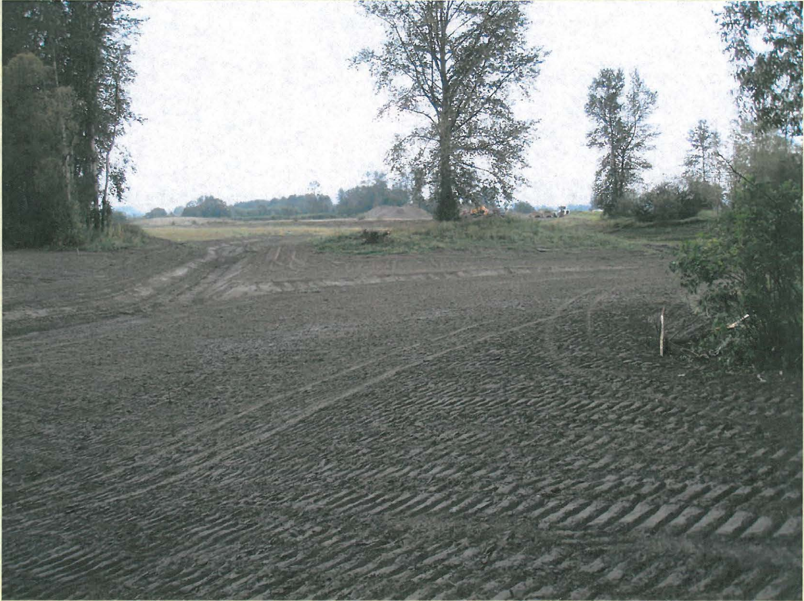
Nookachamps Mitigation Bank during construction
