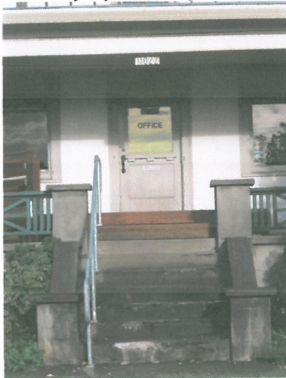
New Entryway w/ Railing:
