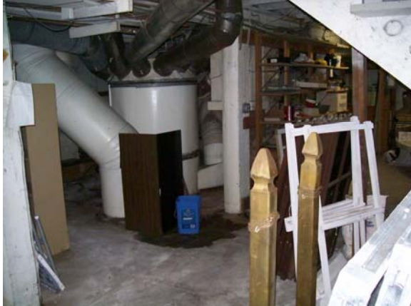
Basement/ Furnace (Before):
