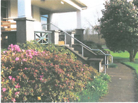
New Exterior Railing:
