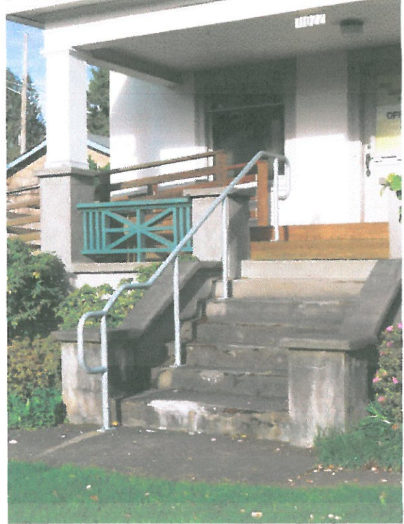
New Exterior Railing:
