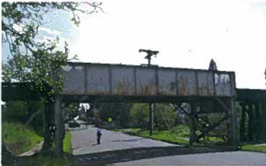
The existing freight rail trestle over Lake Road limits the height of vehicles using the road. A future TriMet light rail bridge will be placed alongside it. The passages underneath these bridges should be designed for pedestrian comfort.
