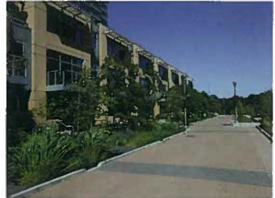
Pedestrian-oriented street with stormwater planters
