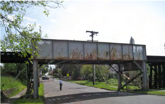
The existing freight rail trestle over Lake Road limits the height of vehicles using the road. A future TriMet light rail bridge will be placed alongside it. The passages underneath these bridges should be designed for pedestrian comfort.
