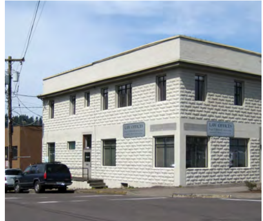
Numerous historic structures help define the character of downtown Milwaukie.
