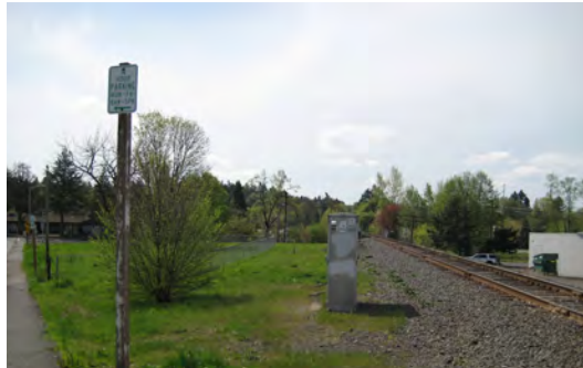
The Triangle site will be the location of a future MAX station, with double tracks to the left of the existing rails in this photo. Comfortable, clear pedestrian access to and from the station will help support the future South Downtown.
