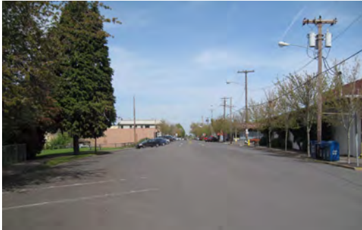
View looking north on Main Street, showing excess paved area and angled parking. Large trees at left should be protected if possible. Overhead power lines should be relocated underground.
