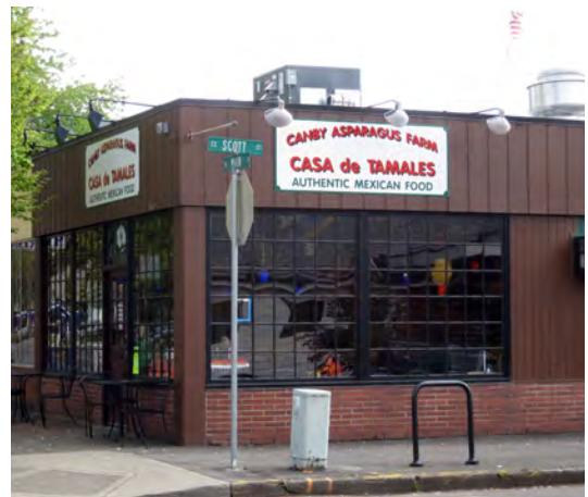
This modest commercial building features generous pedestrian-scaled storefront windows.
