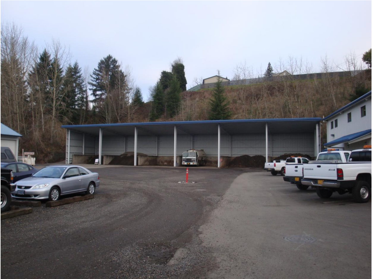
Decant Facility Phase I (Roof structure), October 2010
