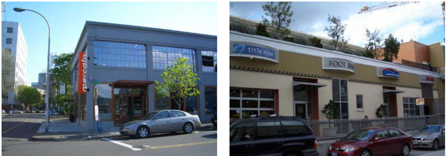
Figure 12. Retrofitted Industrial Buildings with Pedestrian-Oriented Signs
