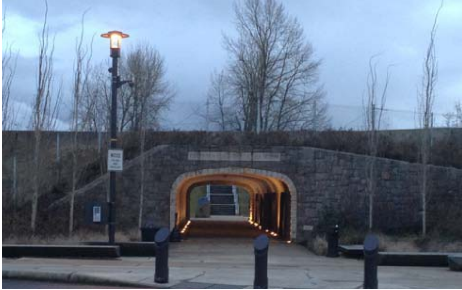
Figure 26. Example of pedestrian undercrossing, Washougal, WA.
