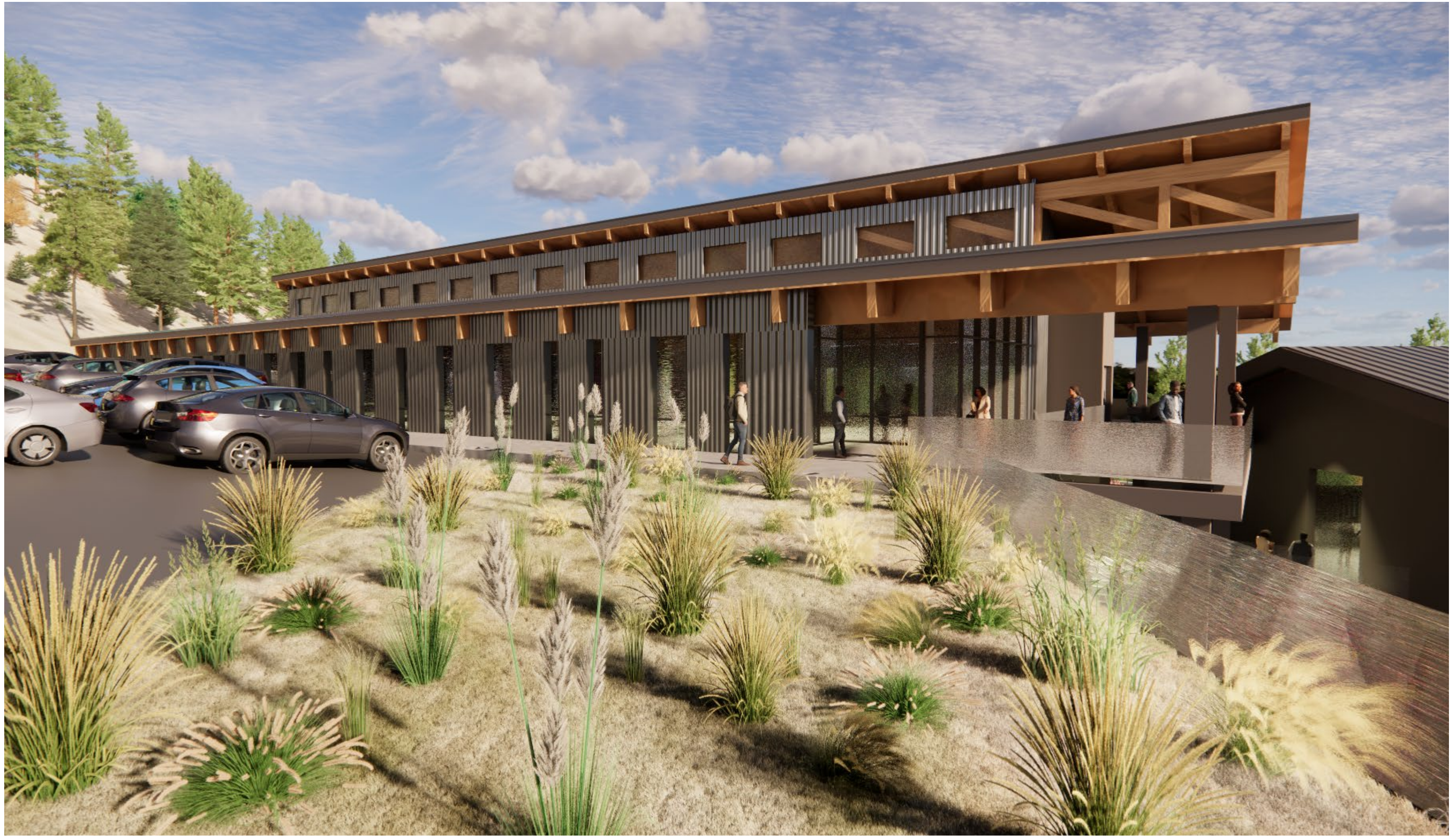
Building C Entry: CLT Structure and Clerestory Daylighting
