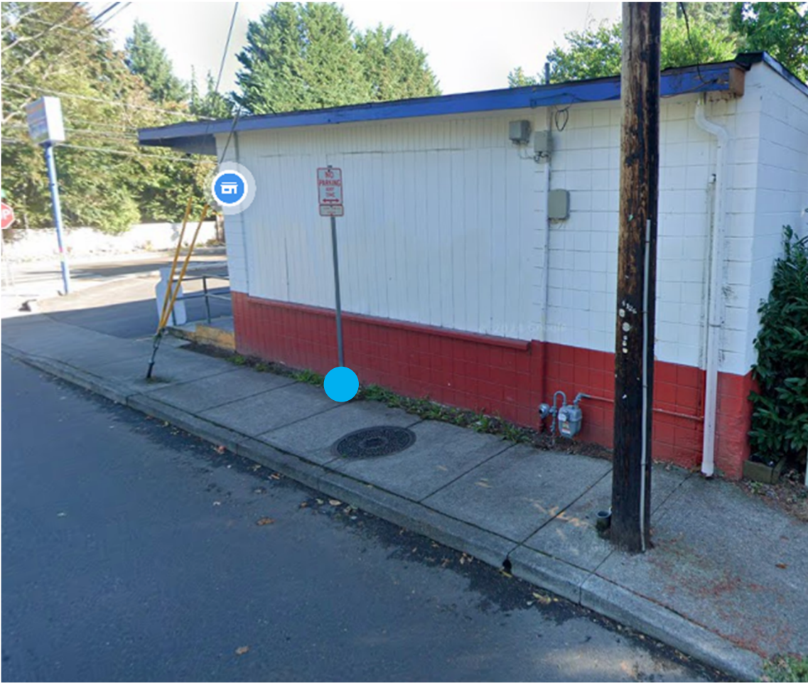
Figure 12: North of Roswell Market (No Parking Tow Away Zone Both Arrows)
