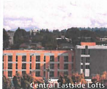
Central Eastside Lofts
