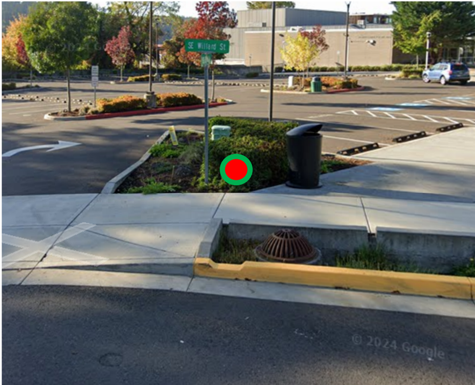
Figure 4: West side of 23 rd , by MHS parking lot approach (No Parking Any Time Right Arrow)
