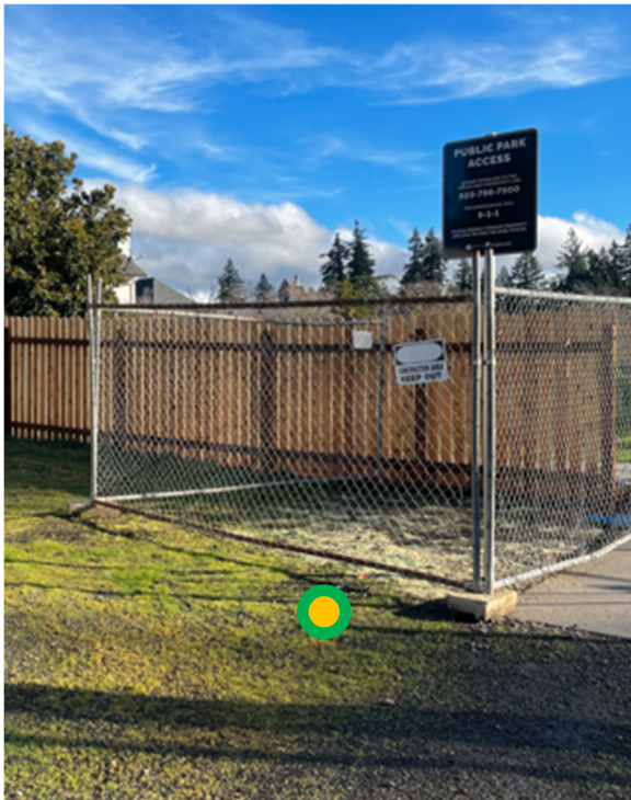
Figure 7: Add "No Parking Fire Lane Left Arrow" sign on single pole on north side of roadway.
