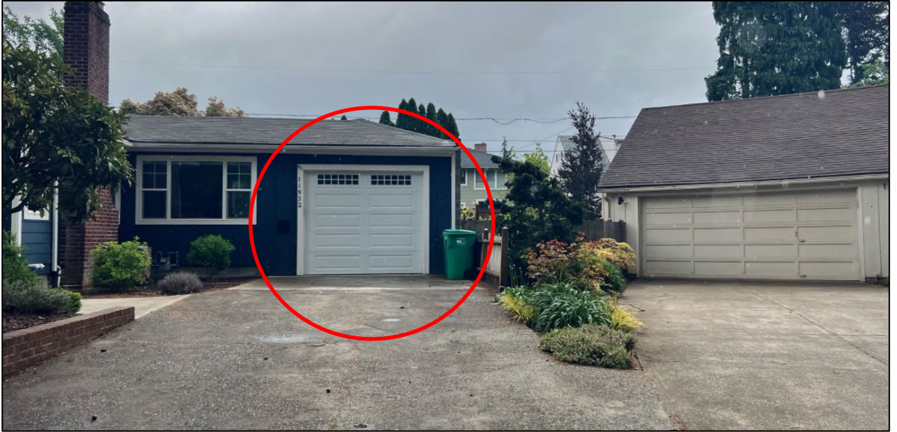
Figure 5. Street view of existing development with location of proposed addition
