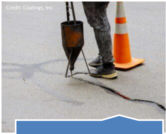
Crack Seal
